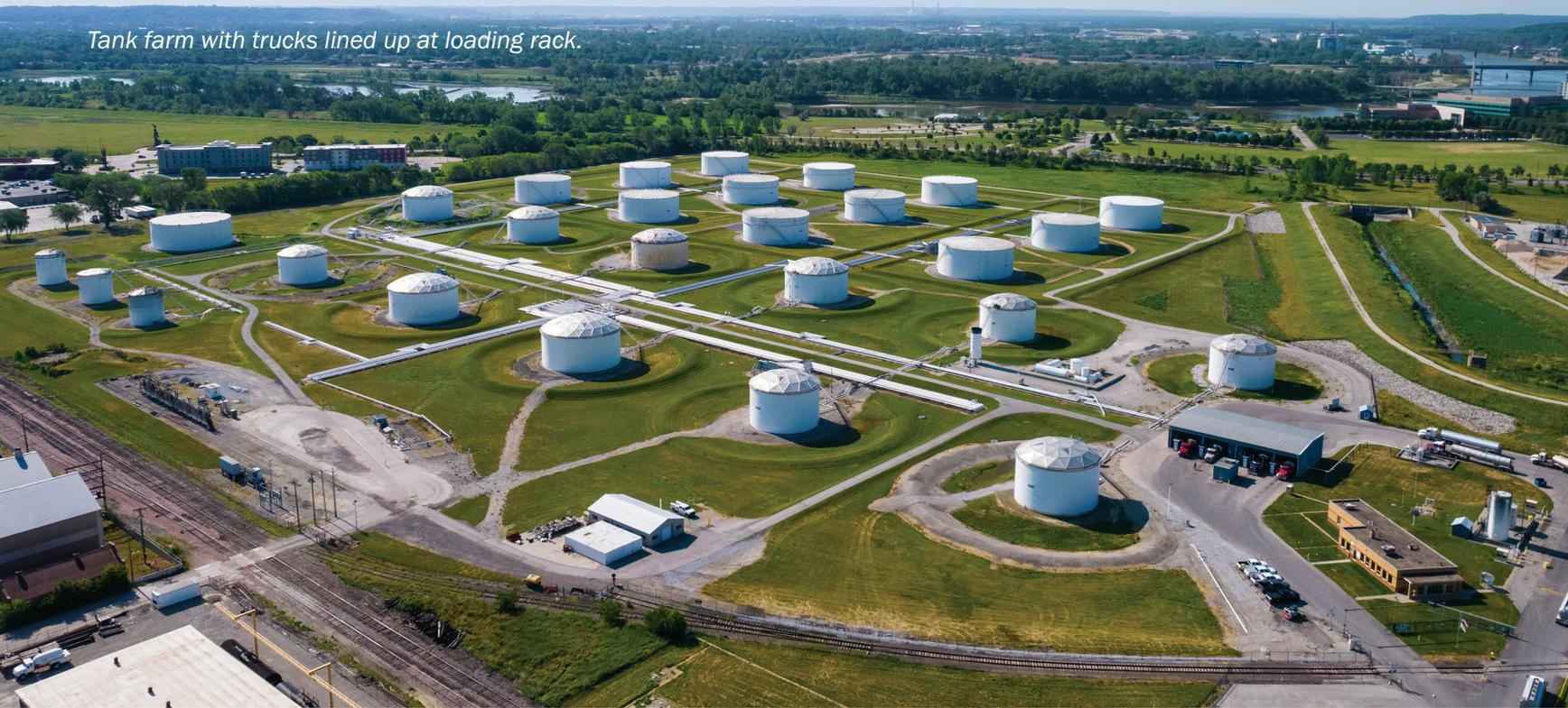
The type of roof is what makes the difference for most storage tanks. Some tanks are built with a solid cone roof with vents along the perimeter. Other tanks may only have a floating roof and some tanks may have an aluminum geodesic dome installed over a floating roof.
